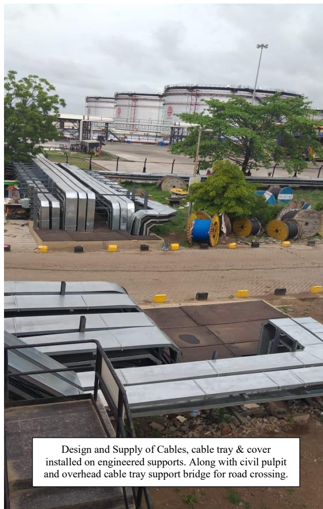
External Cabling System on Cable Trays
