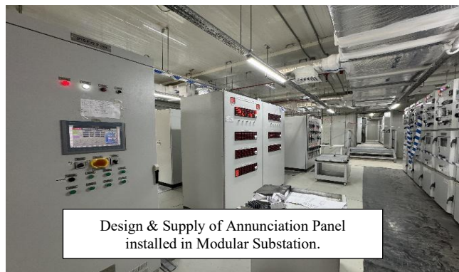
LV Panels and Annunciator Panels
