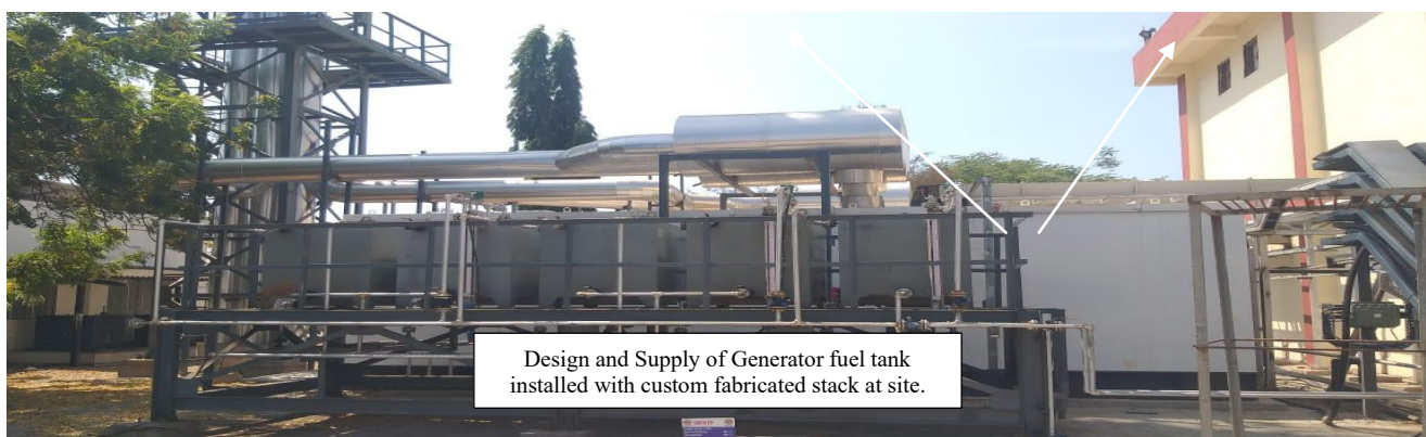
Fuel Tank for Generators
